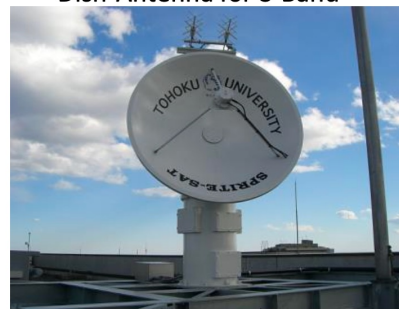
Dish-Antenna for S-Band
