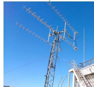
Yagi-Antenna for VHF-band
